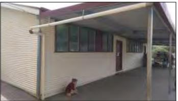
Rooms 1 and 2 were reclad with colourbond steel and any asbestos was removed. The trim was painted in the colours present around the school.
